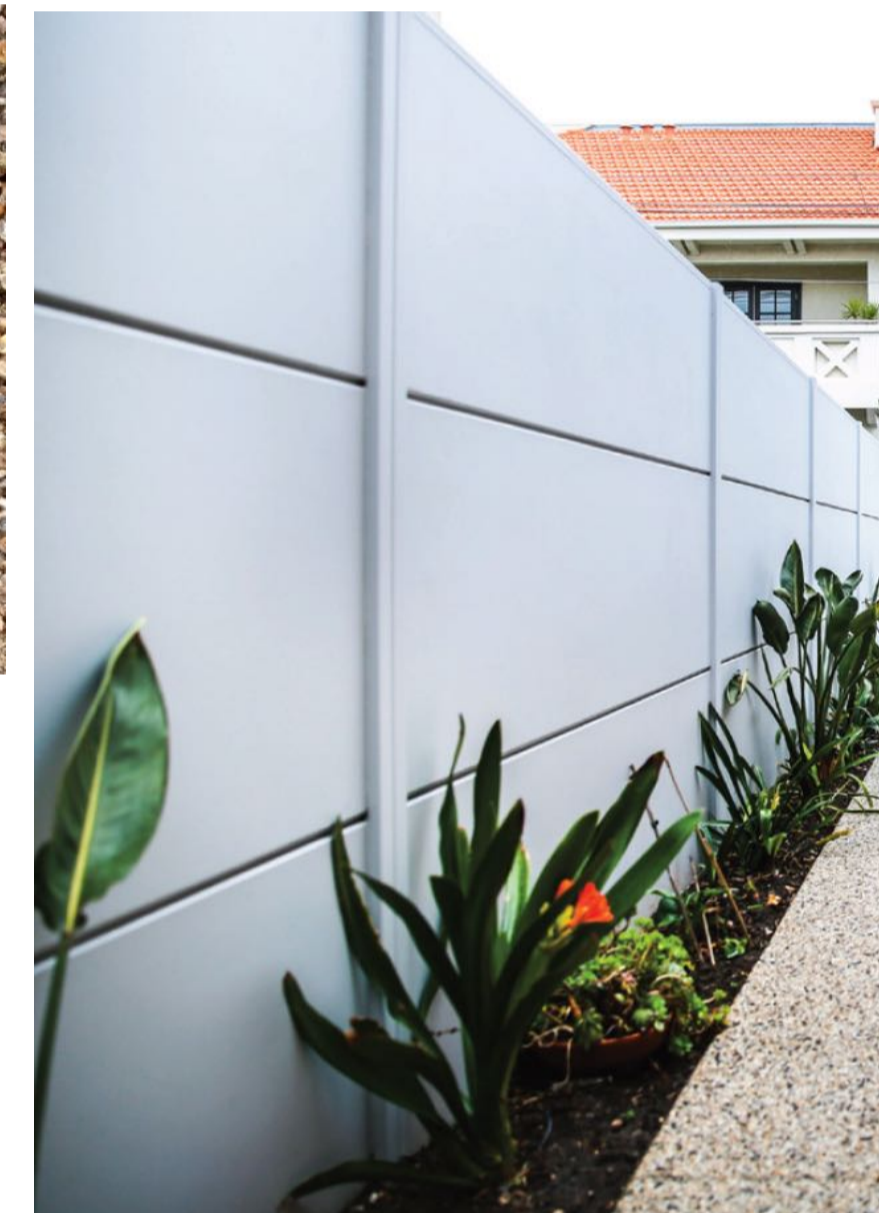
AcoustiMax75 Acoustic Wall, to be 4.5m tall as specified
