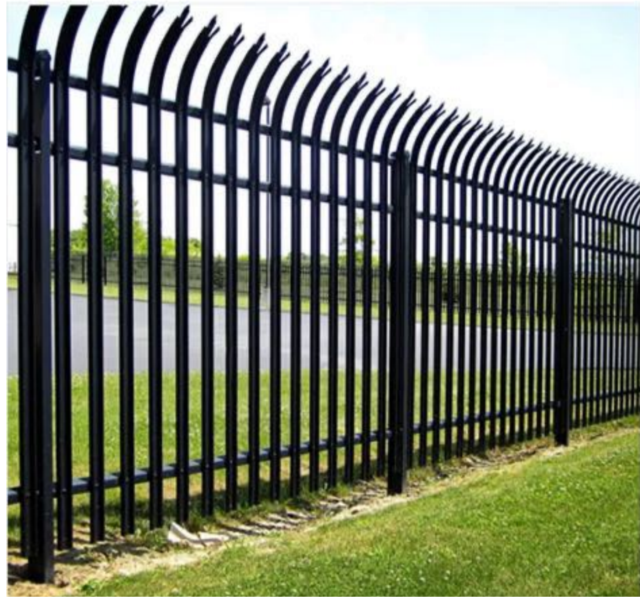
2.1m High palisade fence along southern boundary and Court frontage
