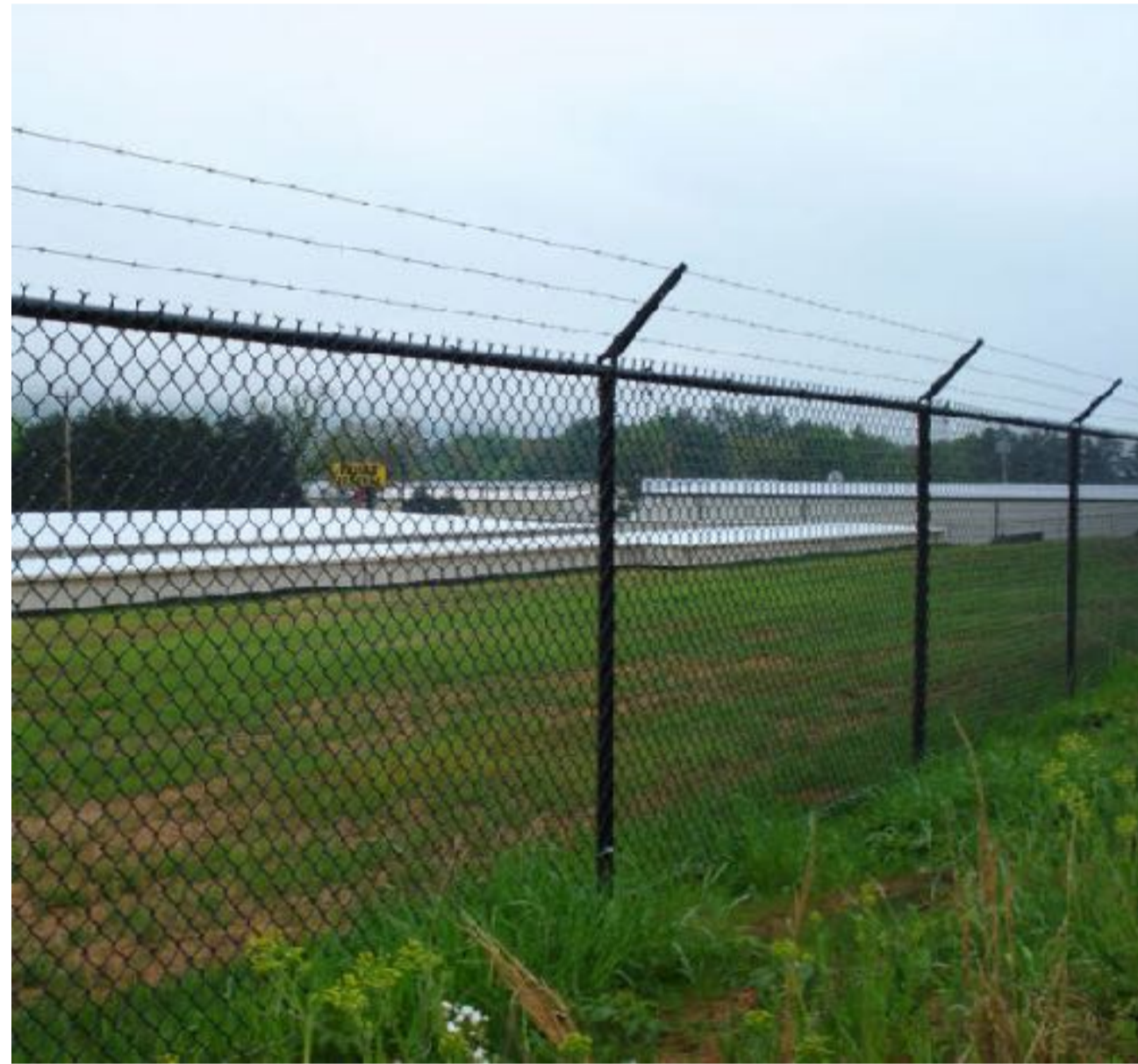
2.1m Chain mesh fence topped with three strands of barbed wire around powerline easement and along eastern boundary of site
