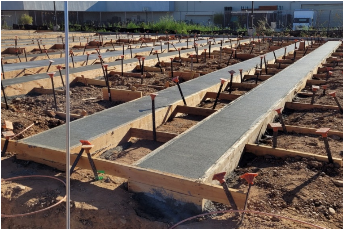
Figure 5: Typical strip footings for Battery and Inverter rows
