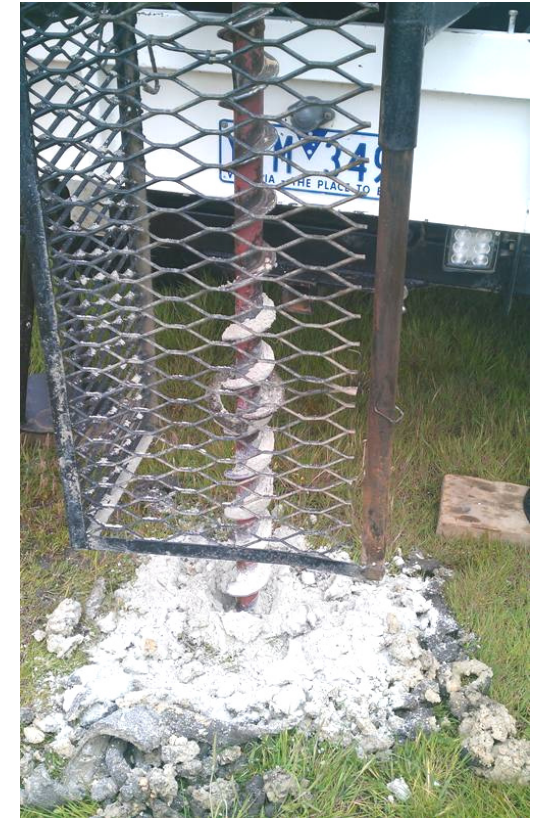
Photo 5: Typical dry material from GW1.
