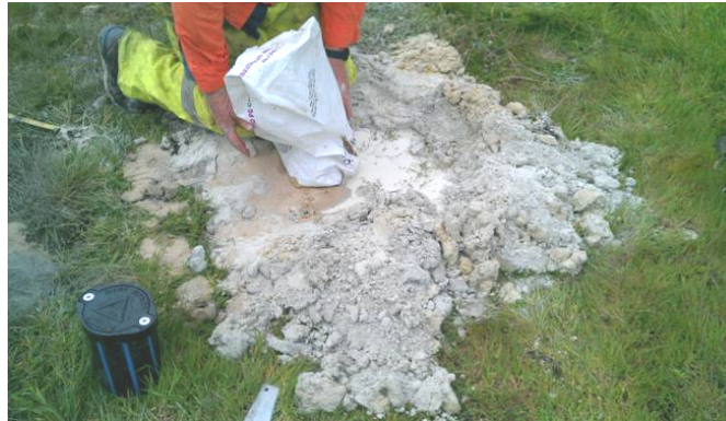
Photo 2: Casing GW1 and packing with sand.
