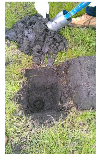
Photo 9: Typical Borehole & excavator material.
