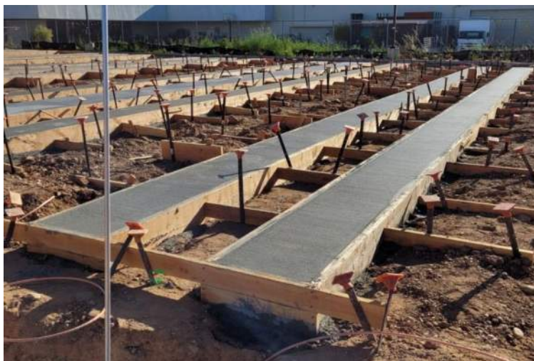
Figure 7: Typical Strip Footings for Battery Cube rows
