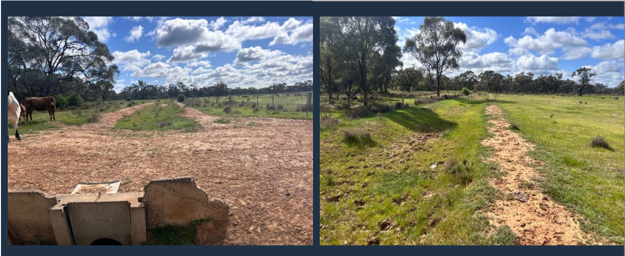
Figure 8-4: Farm Delivery Channel in a state of disrepair and no longer used
