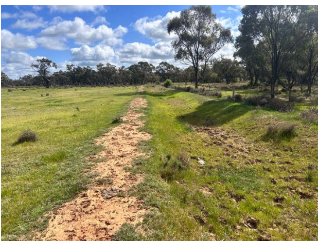
Stockwater surface delivery channel located in south east corner of site
