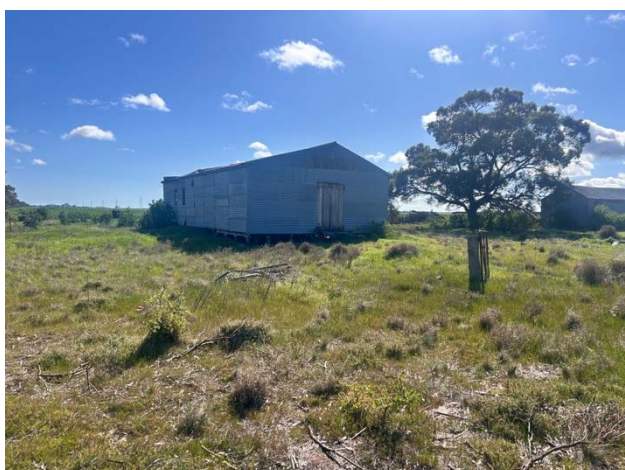
Old Woolshed located on western boundary of site
