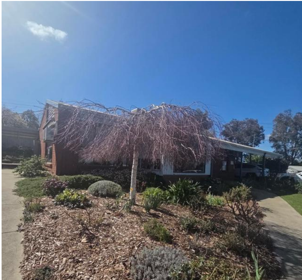
1. View to wellness centre (previous used as a dwelling) nominated for demolition to necessitate the new ELC works.
