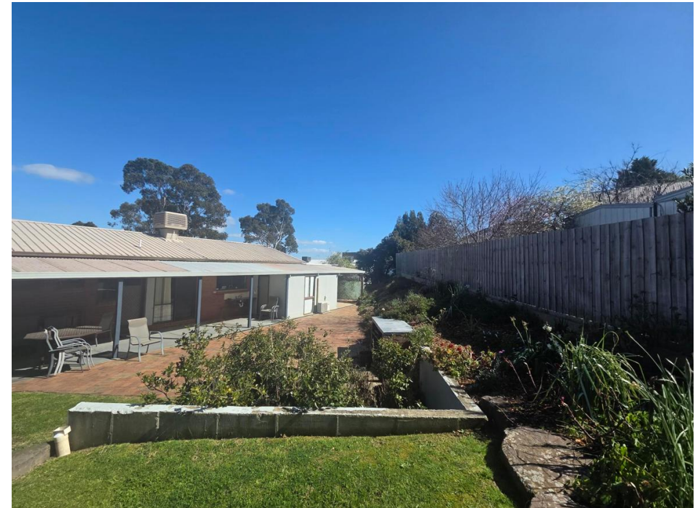
2. View along northern boundary, looking west from north-east corner of the Site. The image illustrates the level change and relationship between the proposed ELC outdoor play area and adjoining residential land at 5 Sulky Court (and beyond). The existing timber paling fence is nominated for retention.
