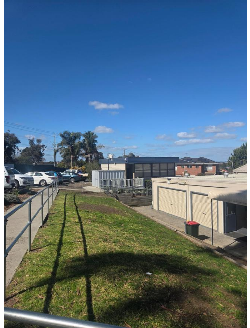
6. View to existing Block D and portable (looking east), with existing level change illustrated.
