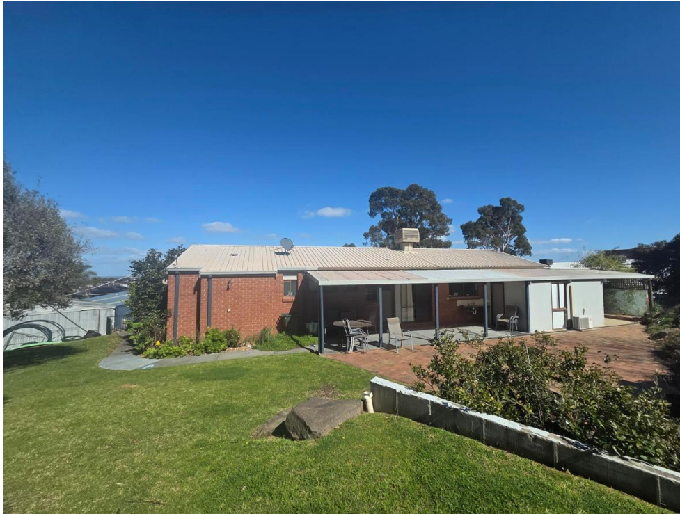
3. Looking south toward the rear of the existing wellness centre building.
