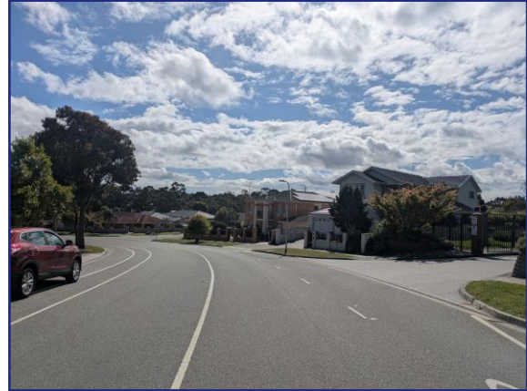
Figure 5: Reema Boulevard – view west
