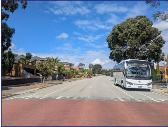
Figure 4: Reema Boulevard – view east
