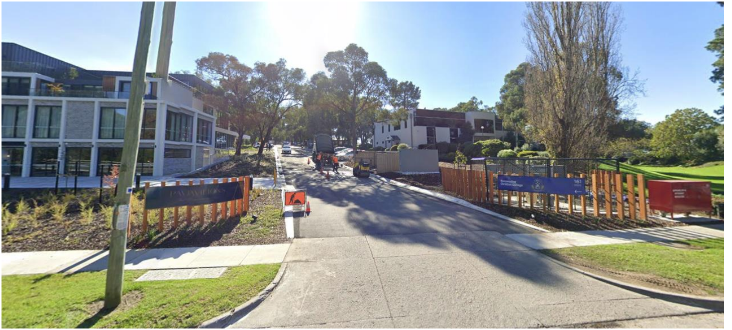
Figure 16 Central Road School entrance, Pavilions Blackburn Lake retirement village adjoining
