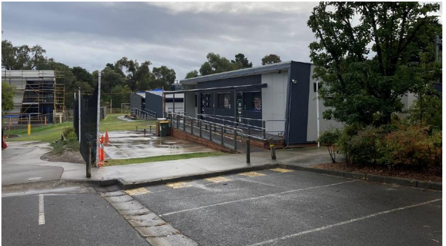
Figure 15 Existing portable classroom building to be demolished
