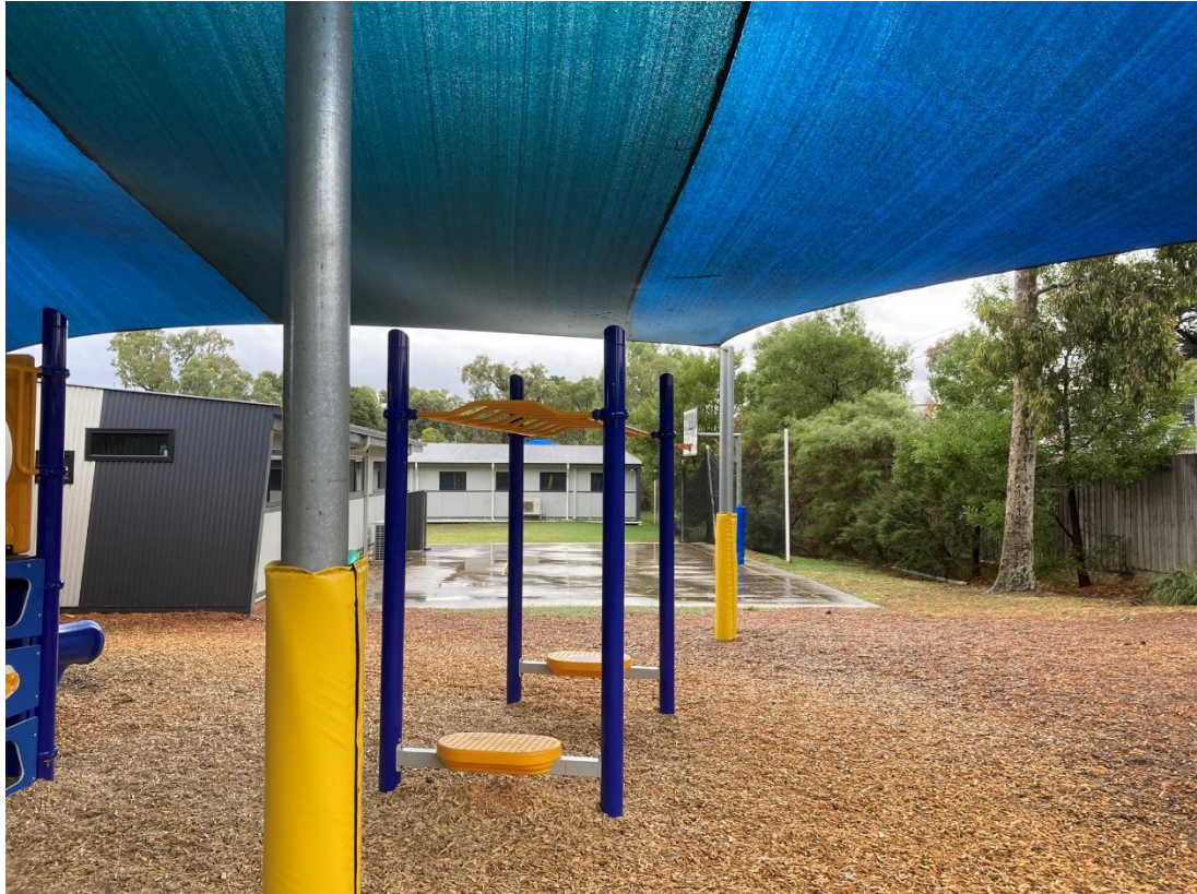
Figure 12: Existing Conditions on northern boundary
