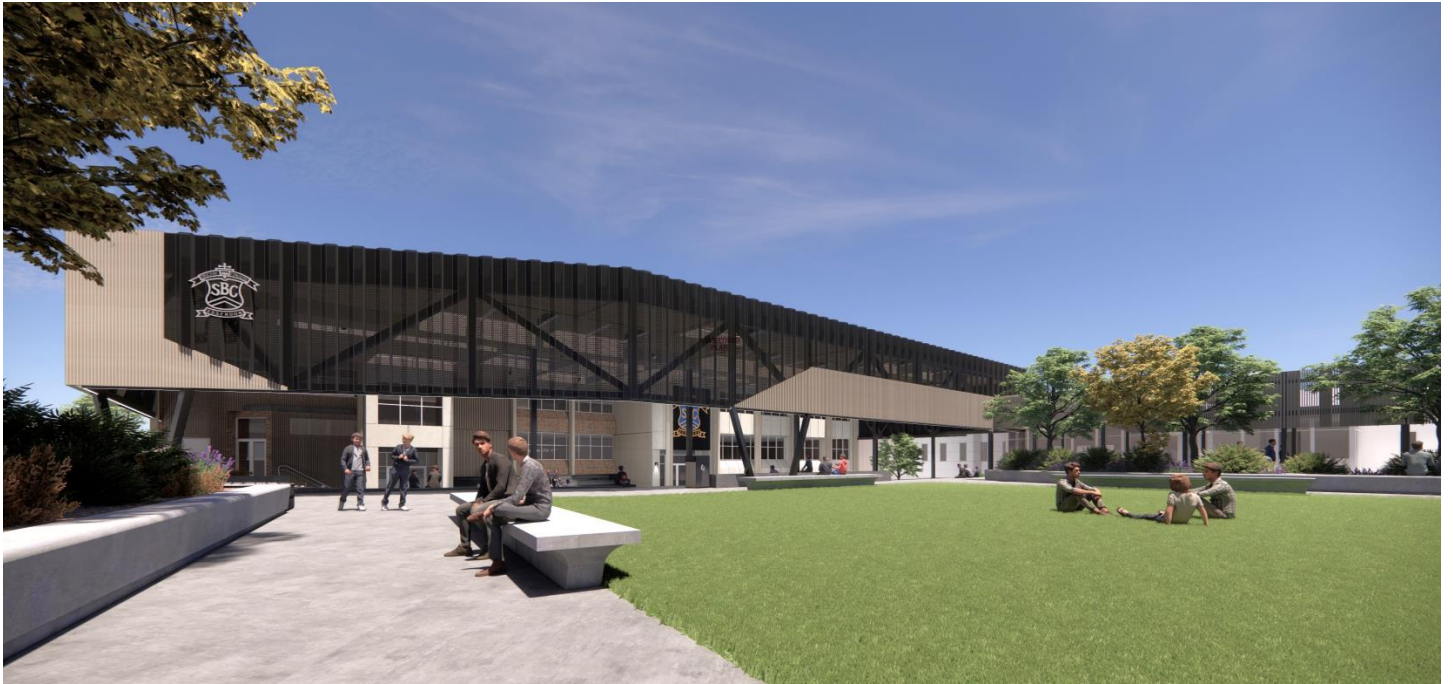
Figure 5 View of the piazza looking towards the Margaret Carey Building, including one of two business identification signs.
