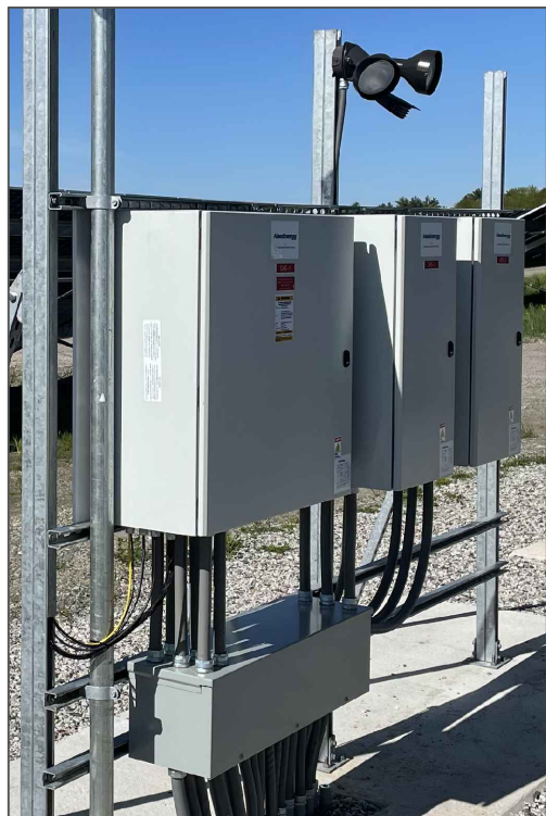
TYPICAL SITE LIGHTING Indicative motion-sensor lights on boards only. As per AS 4282-1997
