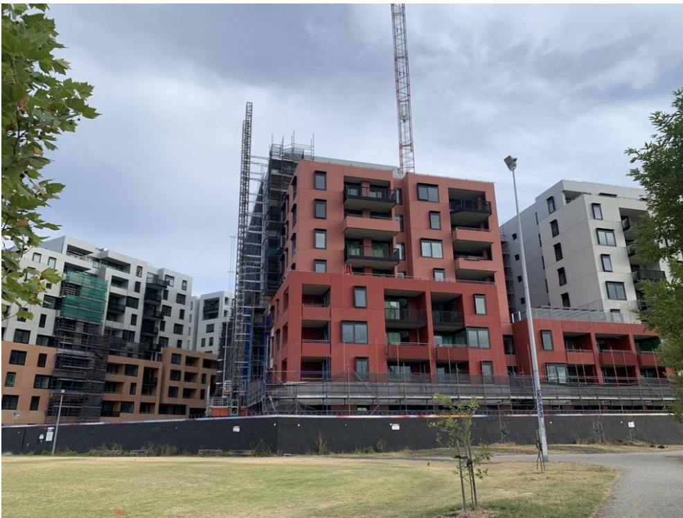
395-411 Albert Street and Subject Site: looking south east from Clifton Park granitic path.
