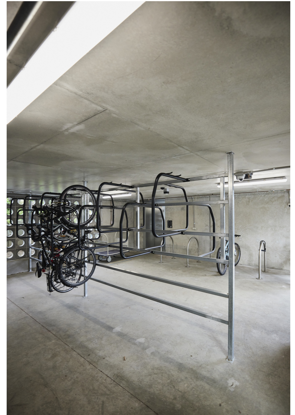
Secure bike parking room at Ferrars & York. Photography by Kim Landy.
