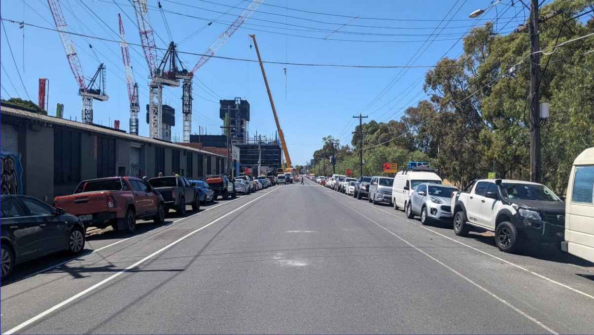
Figure 4: Albert Street – view east
