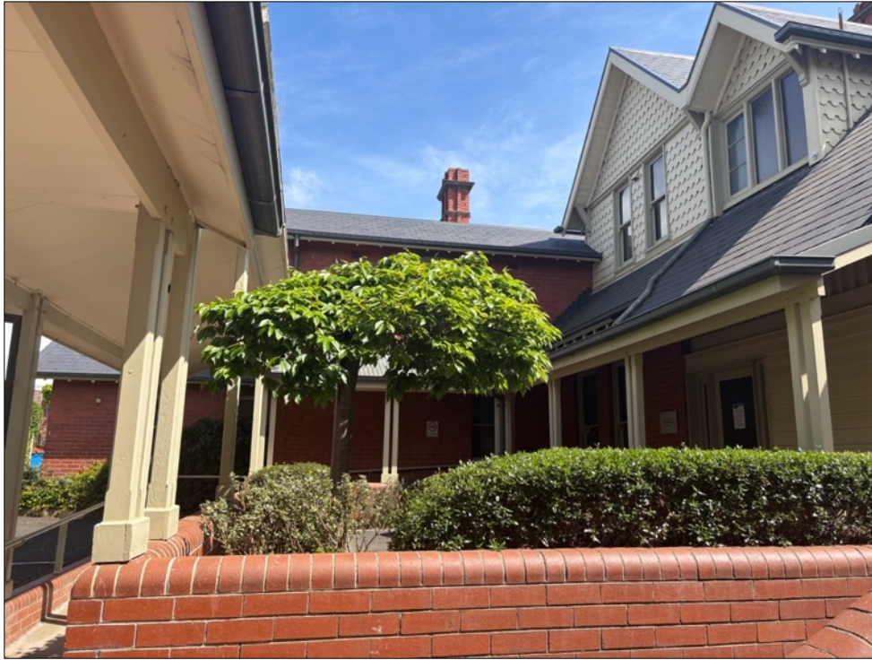
Figure 9 The single storey undercover walkway to the rear of 98 Riversdale Road. Noting the double storey rear wing comprises original fabric.
