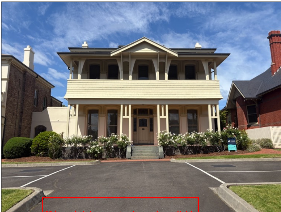
Figure 6 The facade of 100 Riversdale Road, Hawthorn. The original window and door openings are similar to those of 104, while the verandah and balcony date from the early twentieth century.
