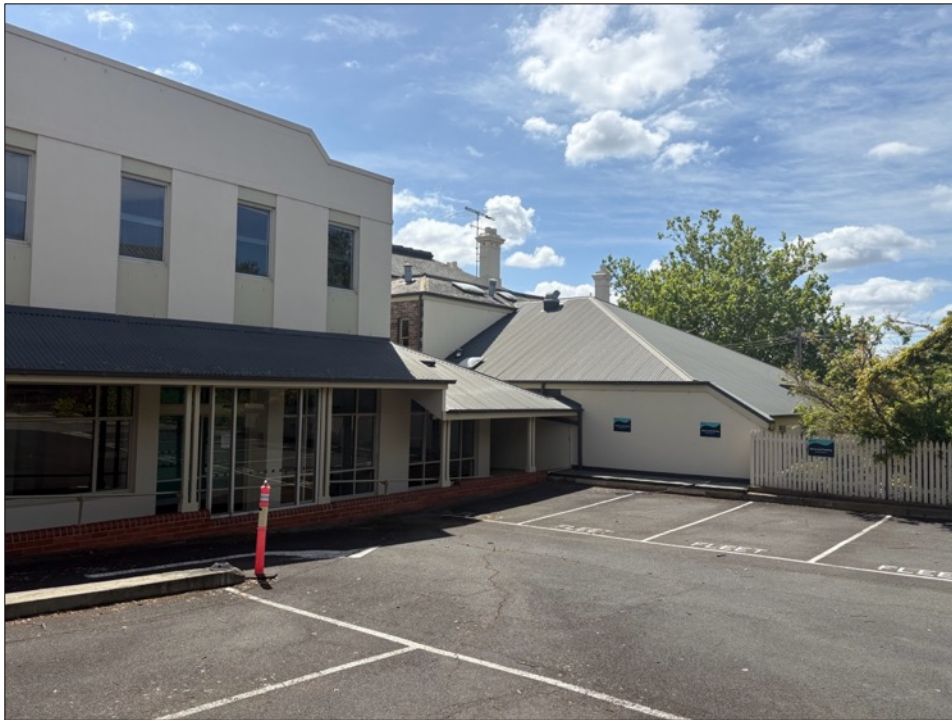
Figure 11 Views to the addition at 104 Riversdale Road. This image also highlights there is a change in gradient to the site.
