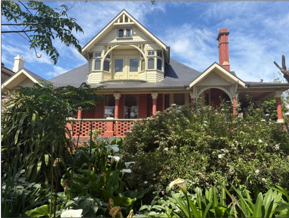
Figure 7 98 Riversdale Road, Hawthorn.
