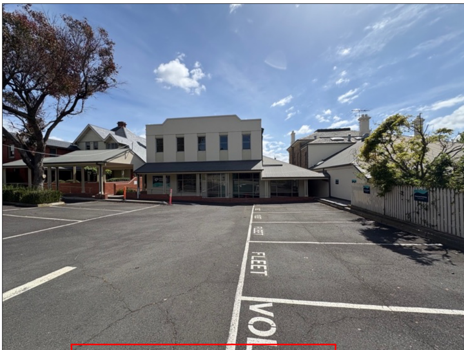
Figure 12 Views to the rear of 100 Riversdale Road, with the double storey rear addition and single storey addition to the south east corner visible.
