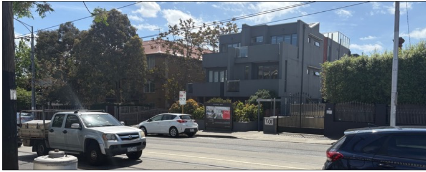
Figure 16 View toward modern apartment buildings on the north side of Riversdale Road, opposite the subject site.
