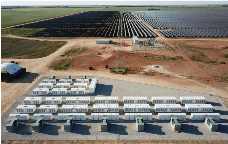
Figure 2-1 Example of 'BESS' and Solar Panel Array
