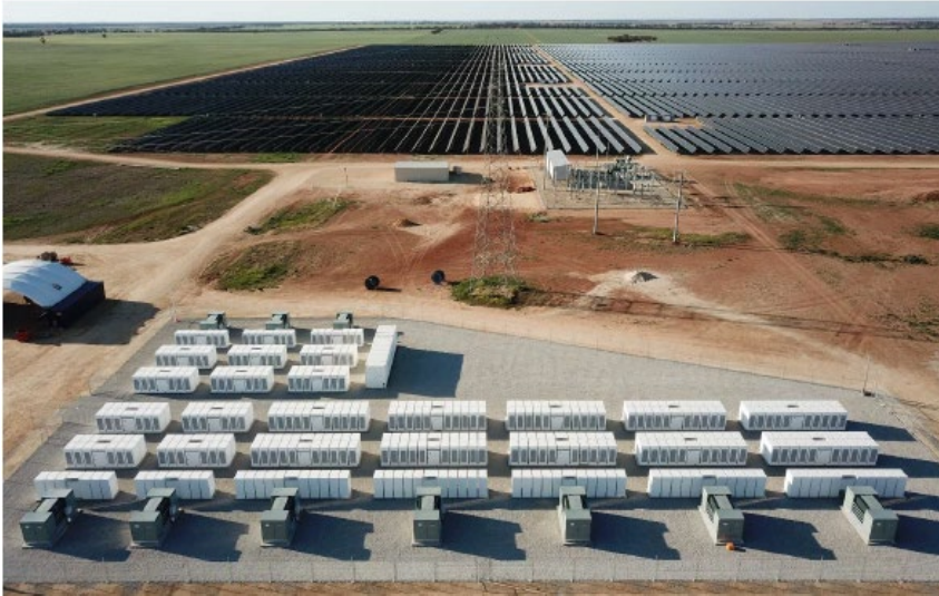
Figure 2-8 Consolidated battery installation example (Source: Edify Energy, 2020)
