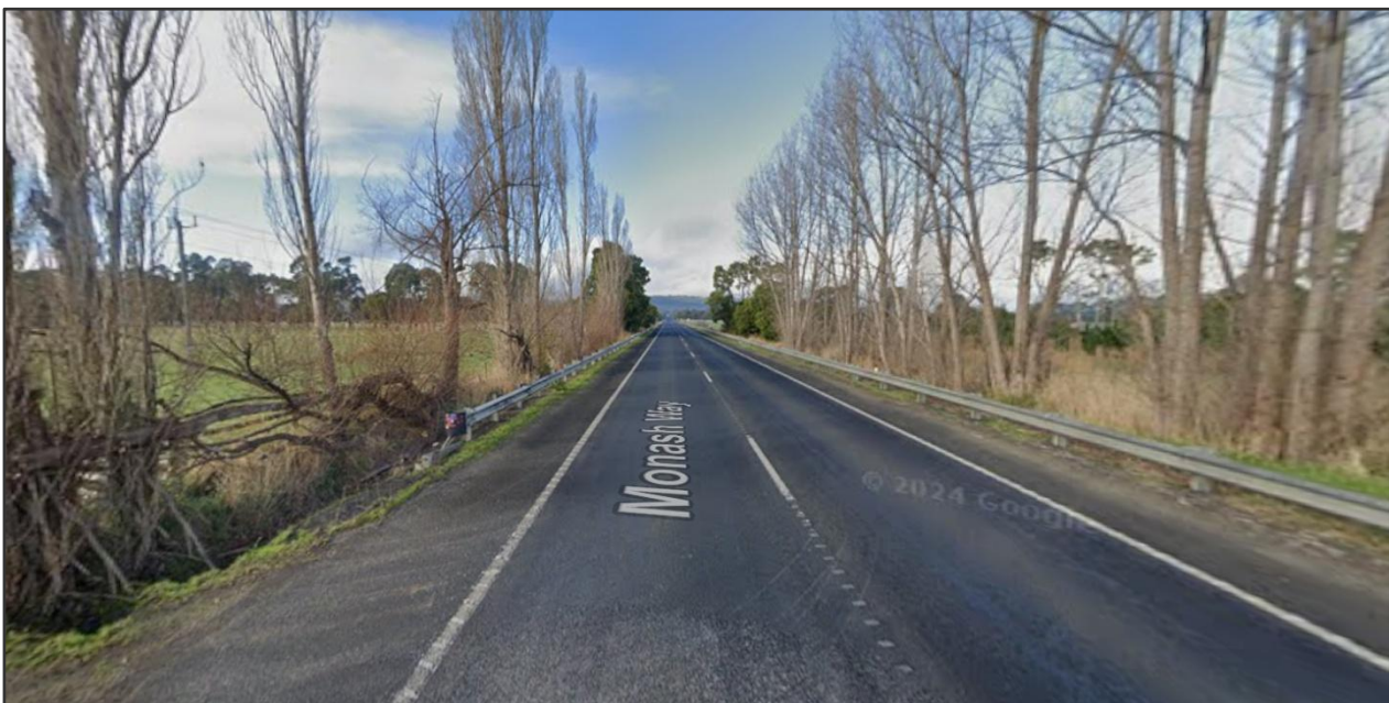
Figure 1 Monash Way Access Sight Line – South
