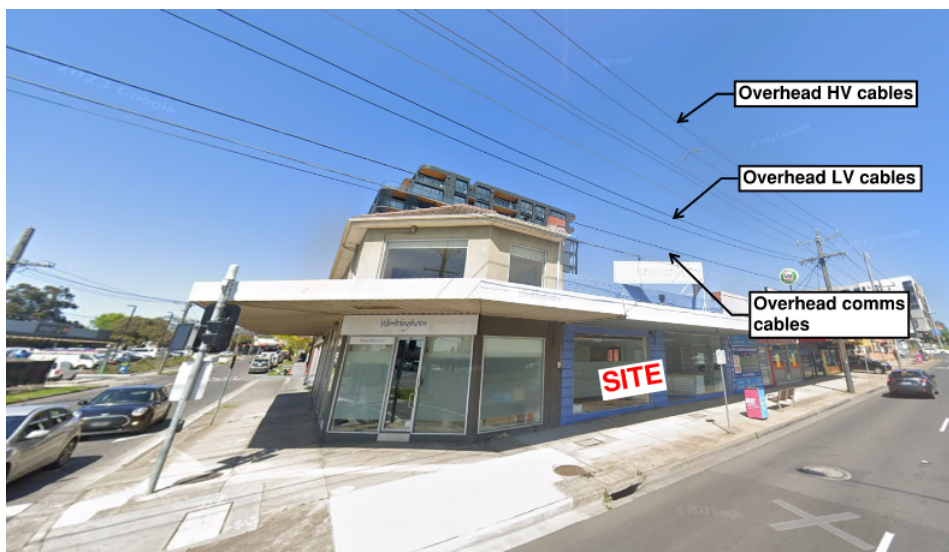
Figure 3 – Overhead Power and Communication Cables
