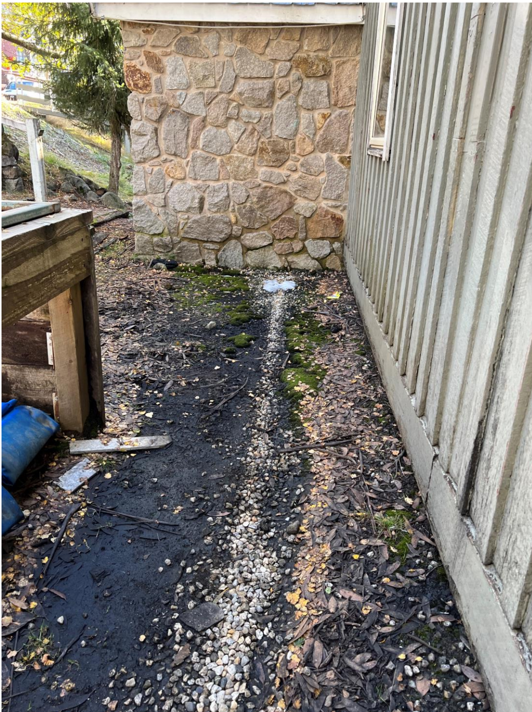
Figure 9 The southern aspect (front) and entryway of Feathertop Lodge. Note the absence of formal drainage and evidence of surface water pooling.
