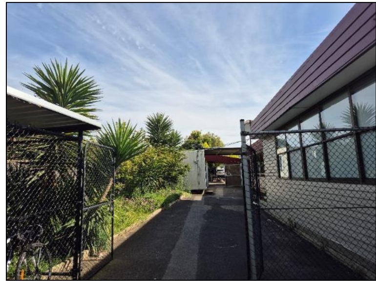
Bitumen walk-way as viewed from south
