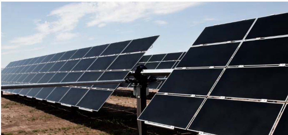
Plate 1. Example of a typical frameless solar array mounted on a single axis tracking system 9
