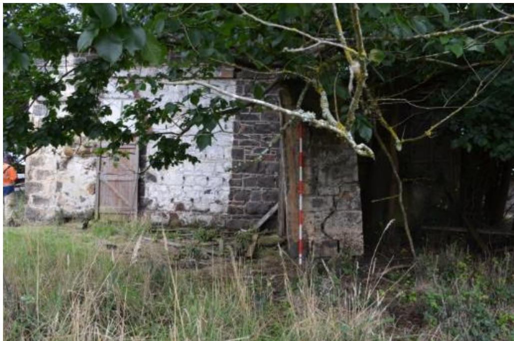
Plate 8: Bath house view west showing newer door added and vegetation growing through structure. Photo A. Wilkinson
