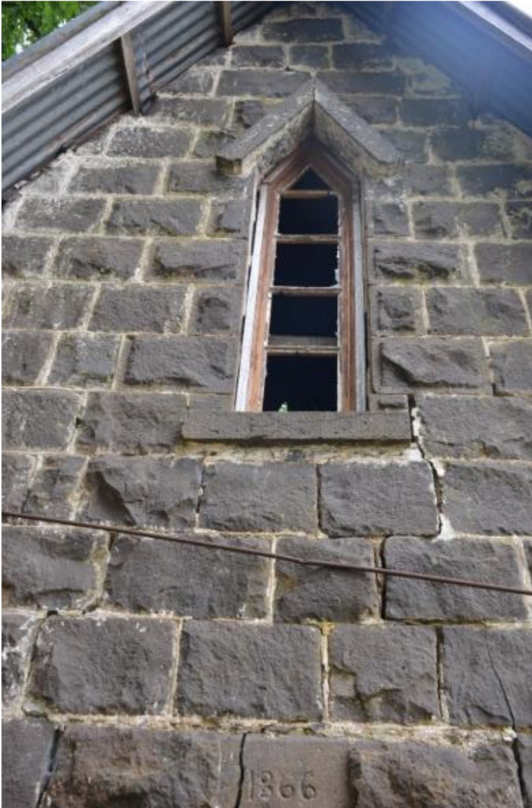
Plate 11: Detail of highlight window and stepped cracking on front of Bath House. View North. Photo A. Wilkinson
