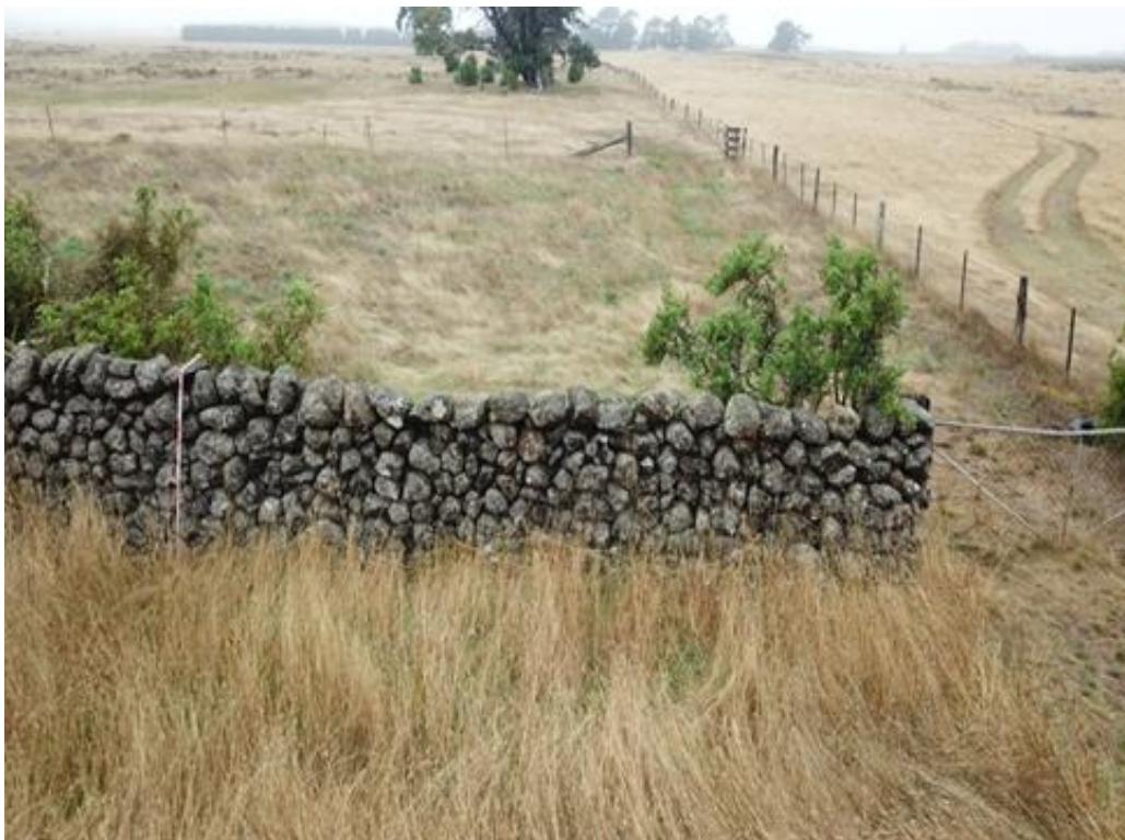
Plate 16: DSW 2 Southern end of DSW-2 showing well-constructed section of wall. Photo A. Wilkinson
