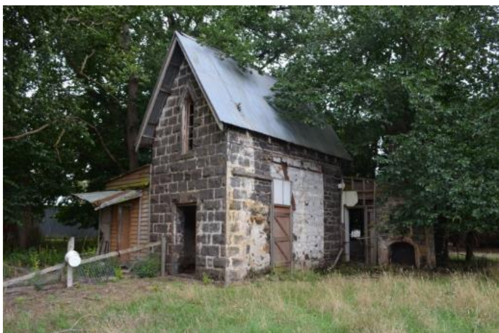
Plate 8: Bath house view west showing newer door added and vegetation growing through structure. Photo A. Wilkinson
