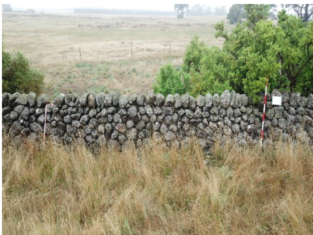
Plate 11: Southern end of DSW-2 showing cope stones (A. Wilkinson 2020).
