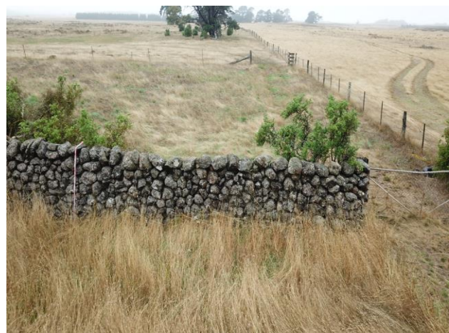
Plate 12: Southern end of DSW-2 showing well-constructed section of wall. (A. Wilkinson 2020).
