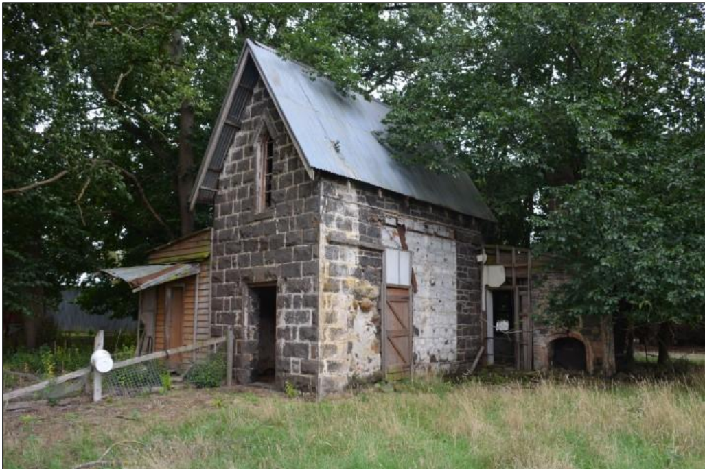
Plate 10: Bath House view west showing newer door added and vegetation growing through structure. Photo A. Wilkinson
