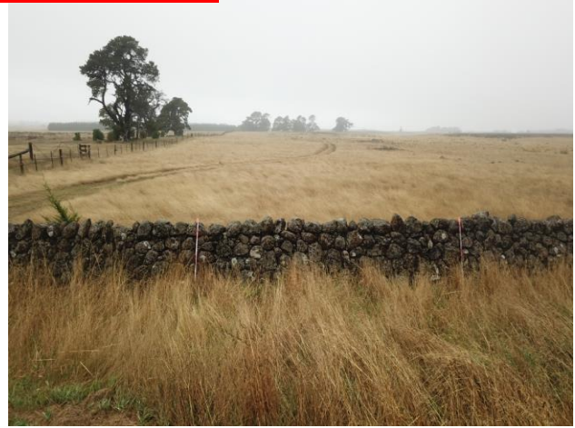
Plate 14: First 30m of DSW-3 showing cope stones in place facing east (A. Wilkinson 2020).
