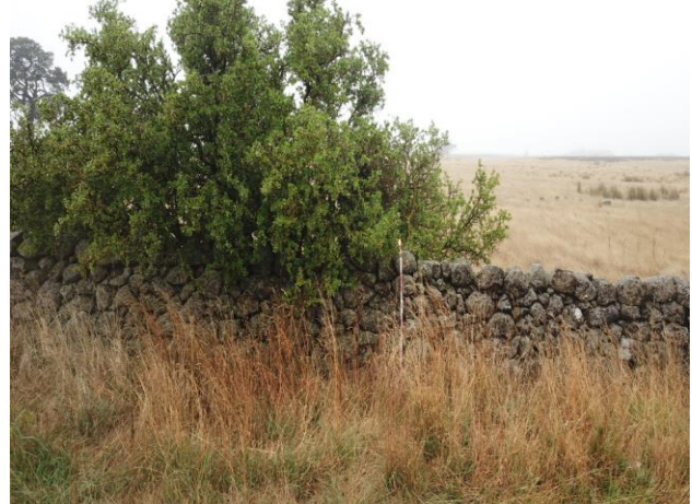
Plate 16: View of section of DSW showing vegetation growth on walls (A. Wilkinson 2020).
