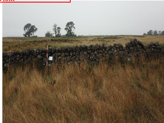
Plate 8: View of DSW-2 showing toppling of cope stones (A. Wilkinson 2020).
