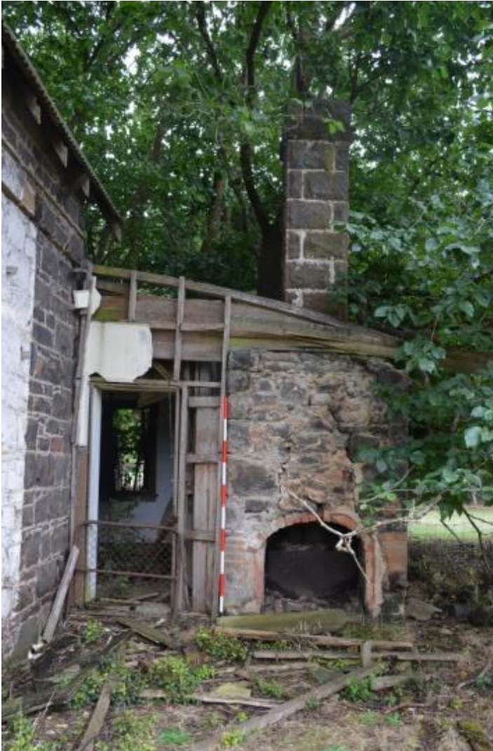
Plate 7: Turkish bath. eastern wall showing hearth used for heating, collapsed door and timber structure, view north. Photo C. De Leuen
