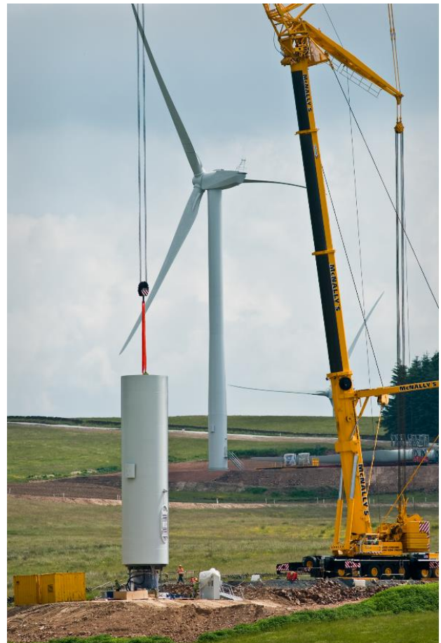
FIGURE 3 EXAMPLE OF TURBINE CONSTRUCTION (SOURCE: WWF)
