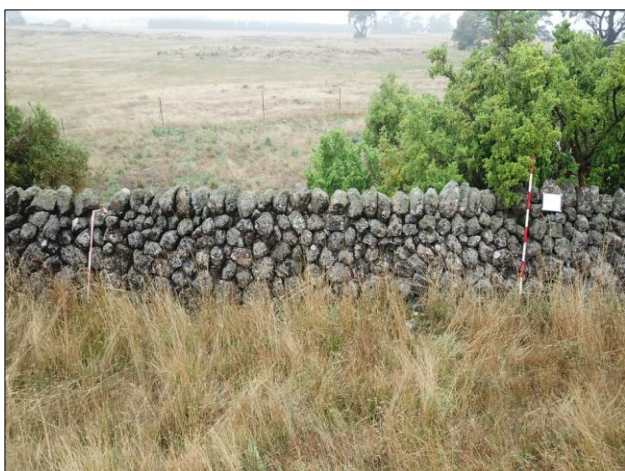
Plate 11: Southern end of DSW-2 showing coping stones (A. Wilkinson 2020).
