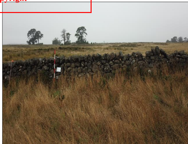
Plate 8: View of DSW-2 showing toppling of coping stones (A. Wilkinson 2020).
