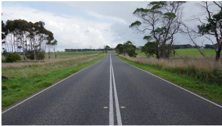
Figure 2-3 Woolsthorpe-Heywood Road, east of Tarrone North Road
