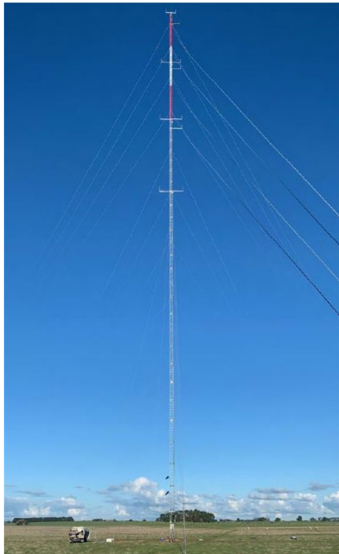
Figure 3-15 Meteorological monitoring mast
