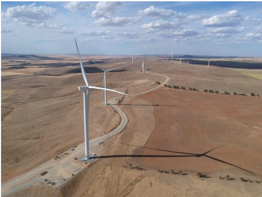
Figure 3-16 Typical Internal Access Road
