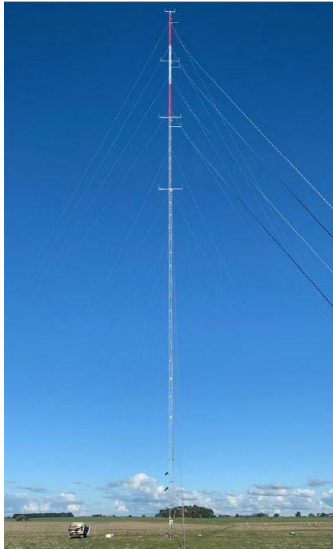
Figure 3-14 Example Meteorological Monitoring Mast
