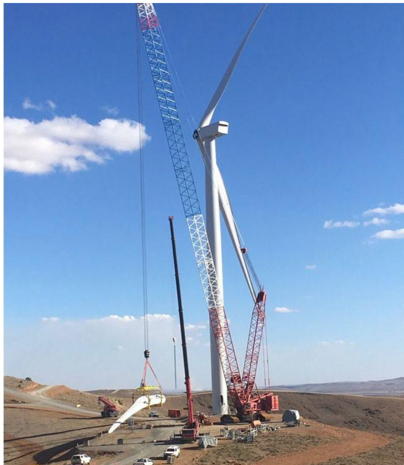
Figure 3-7 A rotor with three blades with the final blade being lifted onto a wind turbine tower
