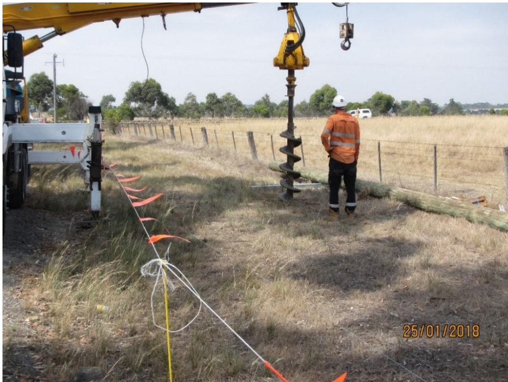
Figure 3: Example of hole being augured via arm from truck (note in this example the roadside vegetation was deemed to be native in places and fencing was set up to keep the truck from the shoulder)
