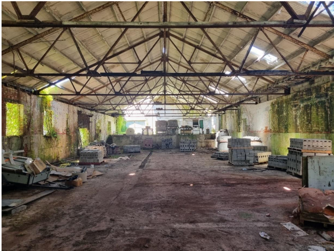
Figure 14: Existing internal structure of the former cheese factory
