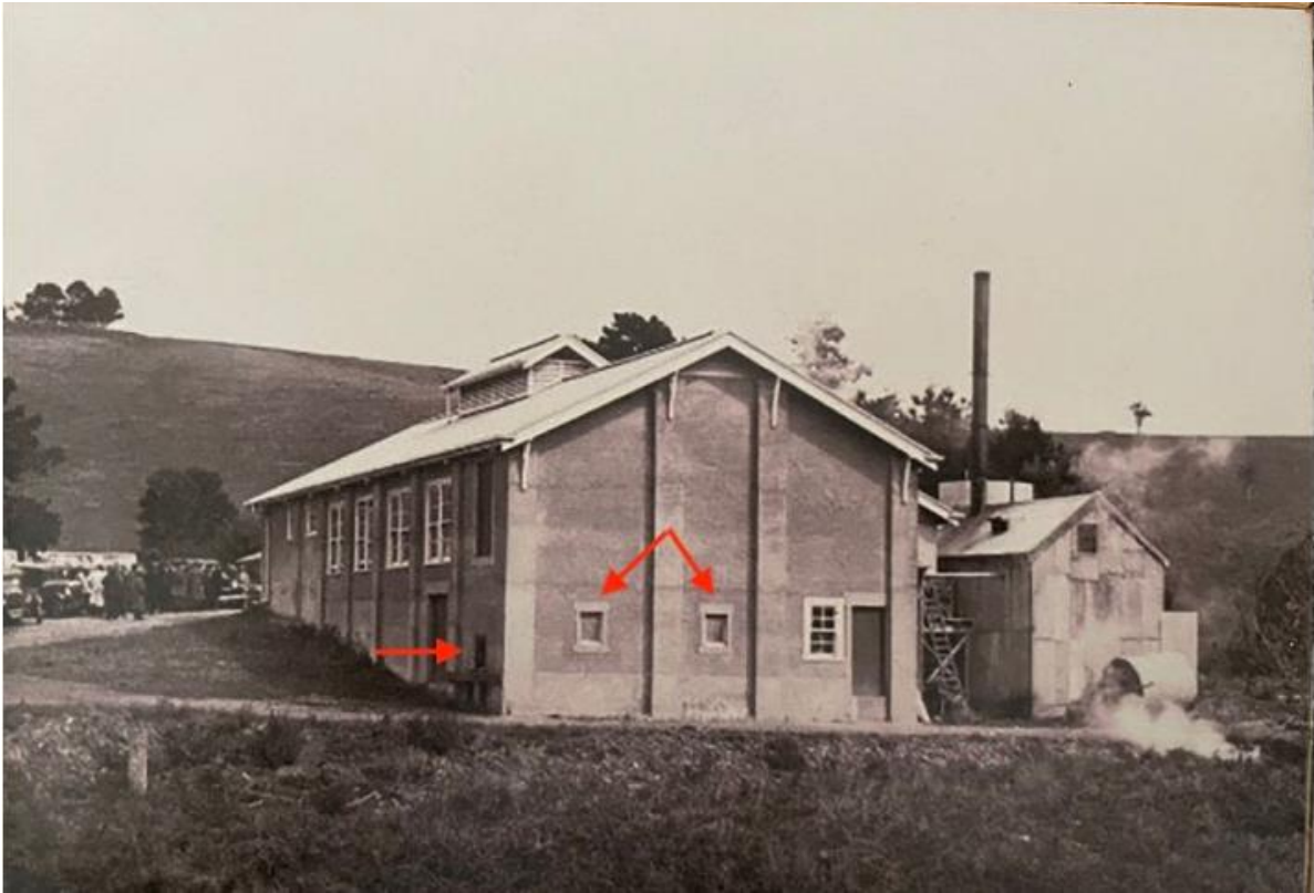
Figure 37: c.1920s/30s image of the former butter factory showing the original openings that will be reinstated.
