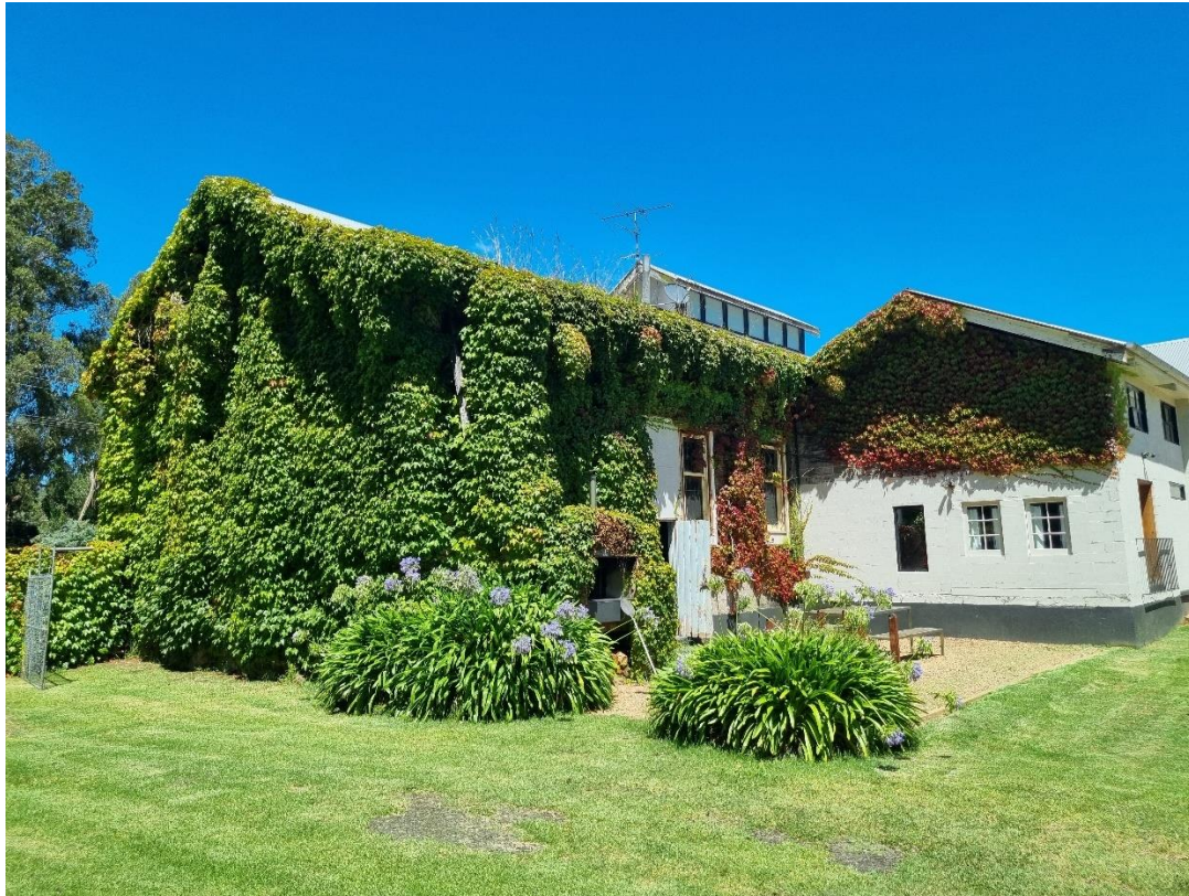
Figure 17: Side (east) elevation of the former butter factory
