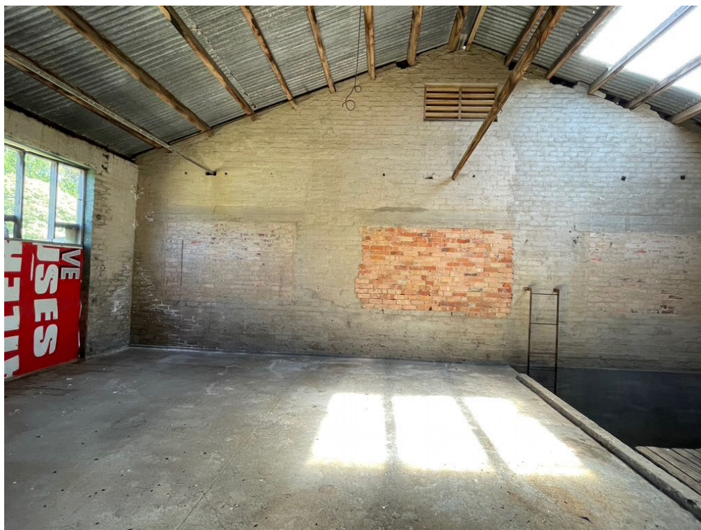
Evidence of bricked-in windows in central wall of western bay.
