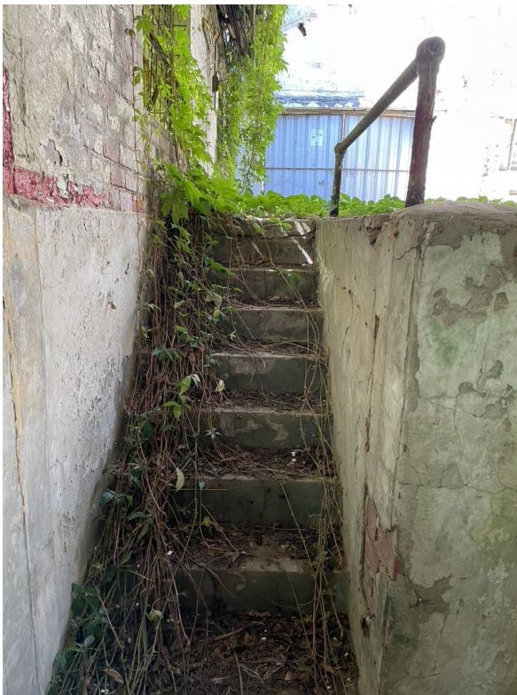
Stair and metal rail at one side of raised platform.
