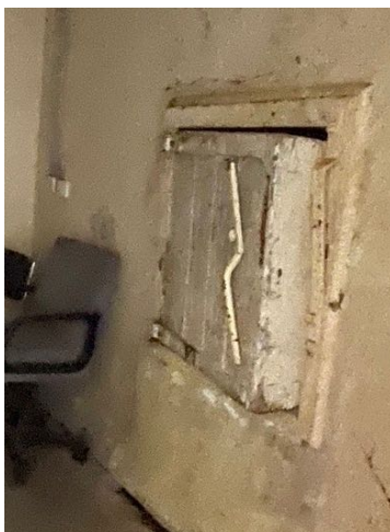
Figure 5: Top: c.1920s/30s image of the former butter factory showing the original openings in the east and front elevation (indicated by added red arrows) that will be reinstated. The lower image shows the original door to the front opening that survives and will be retained.
