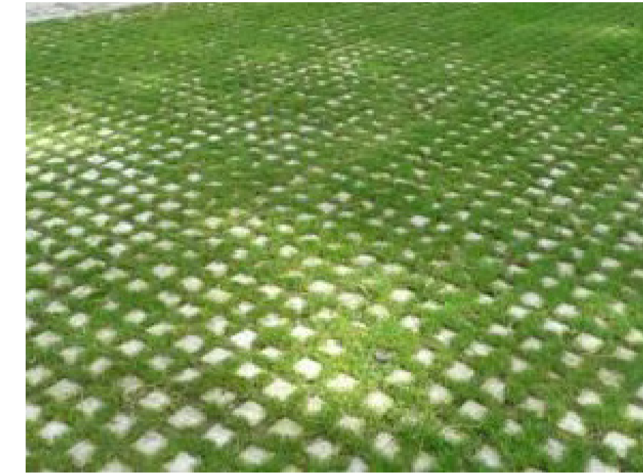
Permeable paving to keep things looking green
