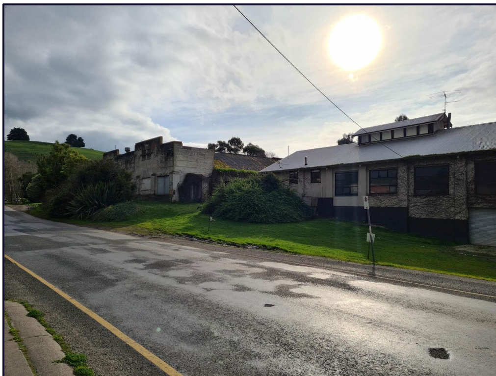
Figure 5: Site photograph looking north-west towards the existing butter and cheese factories.
