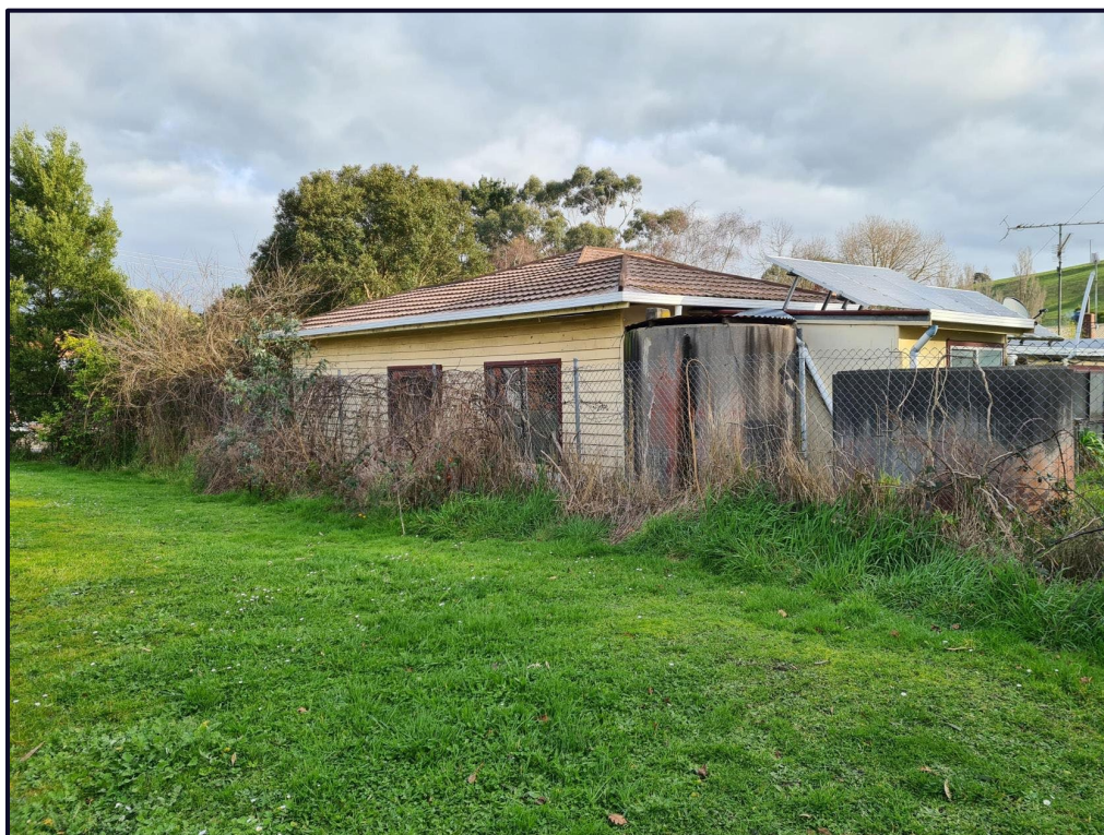
Figure 6: Site photograph of the existing dwelling at 1492 Korumburra-Wonthaggi Road.
