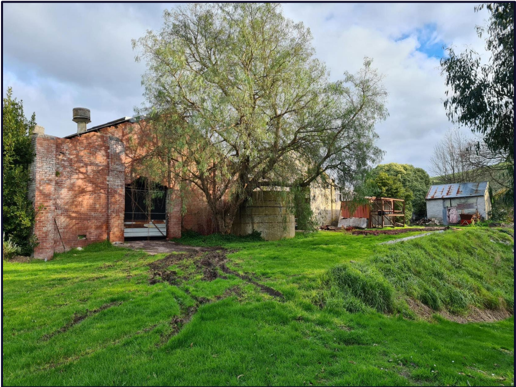
Figure 8: Site photograph looking south-west towards the rear of the existing cheese factory.
