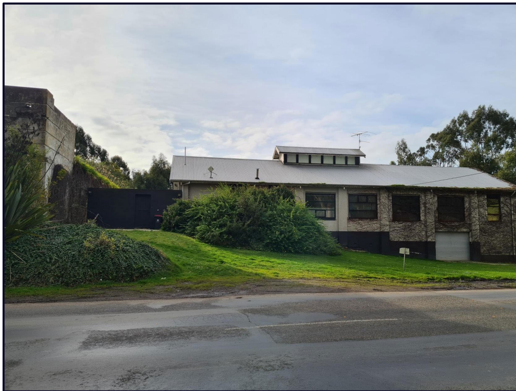
Figure 3: Site photograph looking north towards the existing butter factory.
