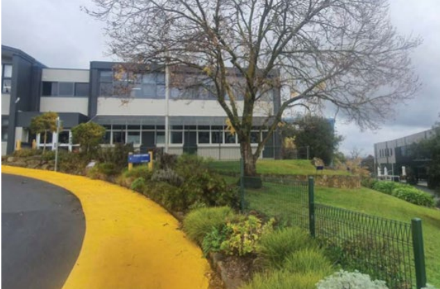
Figure 3.4 Photographs of existing Senior Gertrude Power Building
