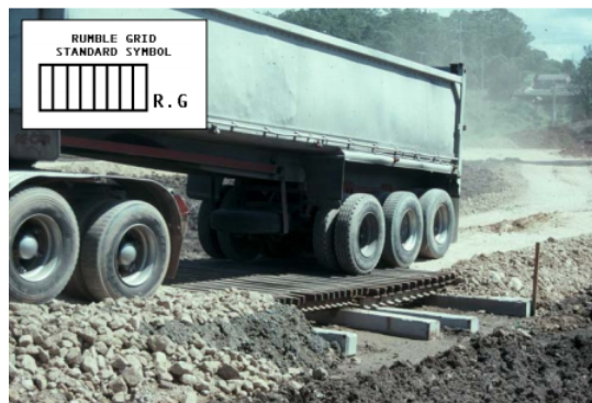
Figure 5.5: Rumble grid (source: EPA Victoria 2004, Publication 960 p.63)
