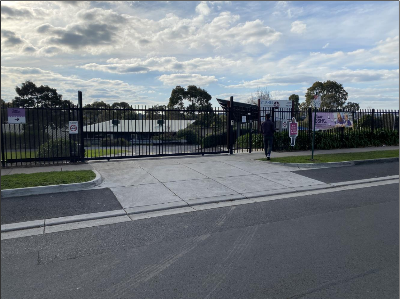
Figure 2 Existing Access Point – Centre Road
