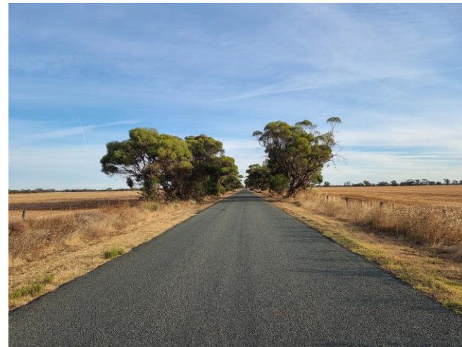
Photograph 8: Denyer Road View North
