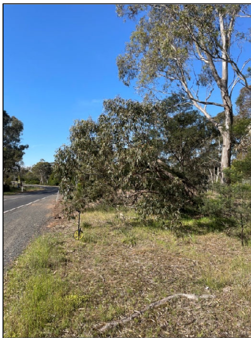
Image 3. Tree 36 at Site 8 will require some minor reduction pruning. Measurement wheel at approximate location of edge of swept path.
