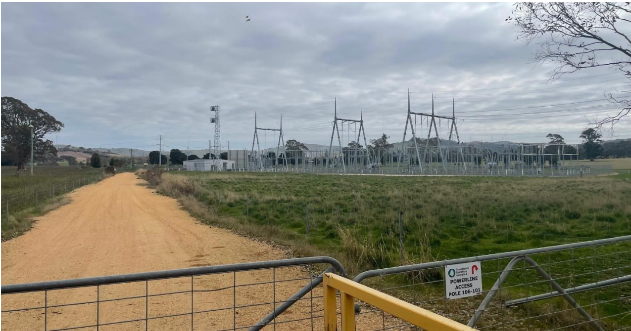
Figure 4. Existing Ararat Terminal Station. DTP Planning Officer, 2023.
