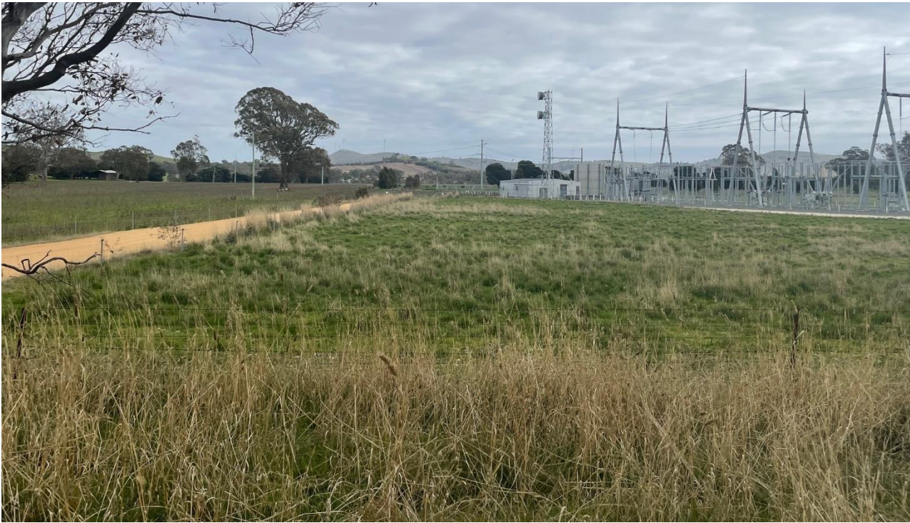
Figure 5. Existing Ararat Terminal Station. DTP Planning Officer, 2023.
