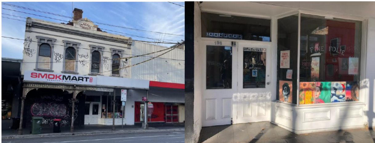
Figure 8: 198-202 Swan Street Building to be retained and refurbished
