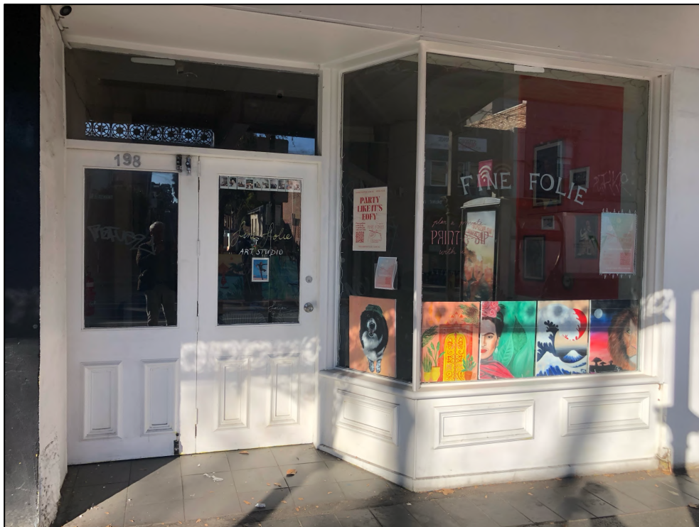
Figure 5 The shopfront of 198 Swan Street. This shopfront, while sympathetic to an early 20 th century appearance, appears to have been reconstructed.
