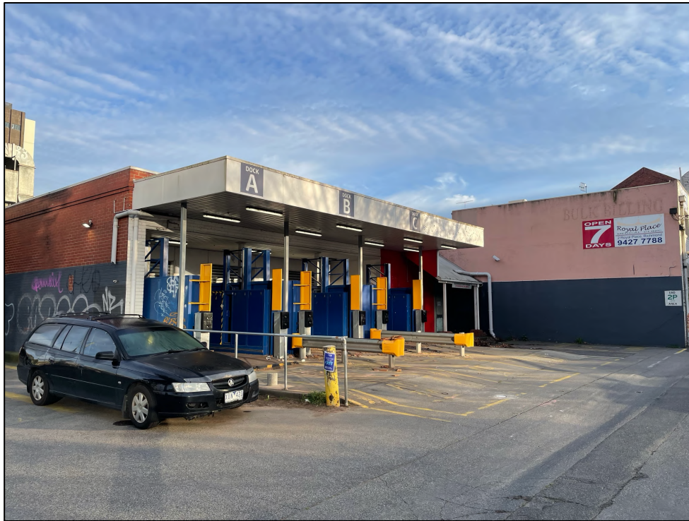
Figure 14 The rear of the development site from the corner of Royal Place and Railway Place.
