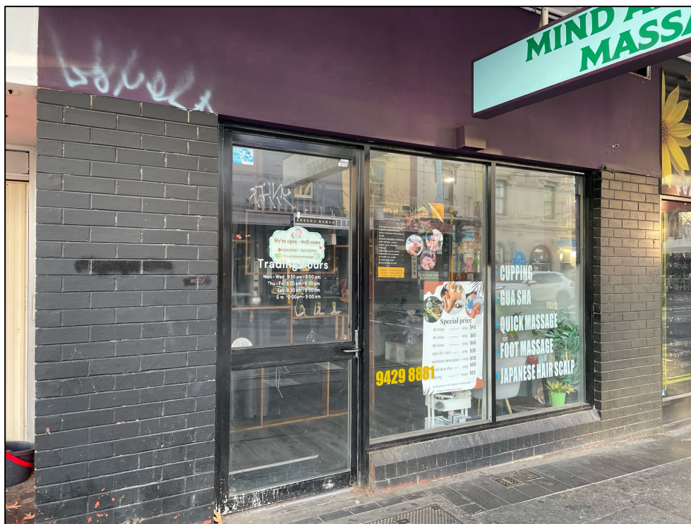
Figure 11 Modern shopfront associated with 192 Swan Street, Cremorne.
