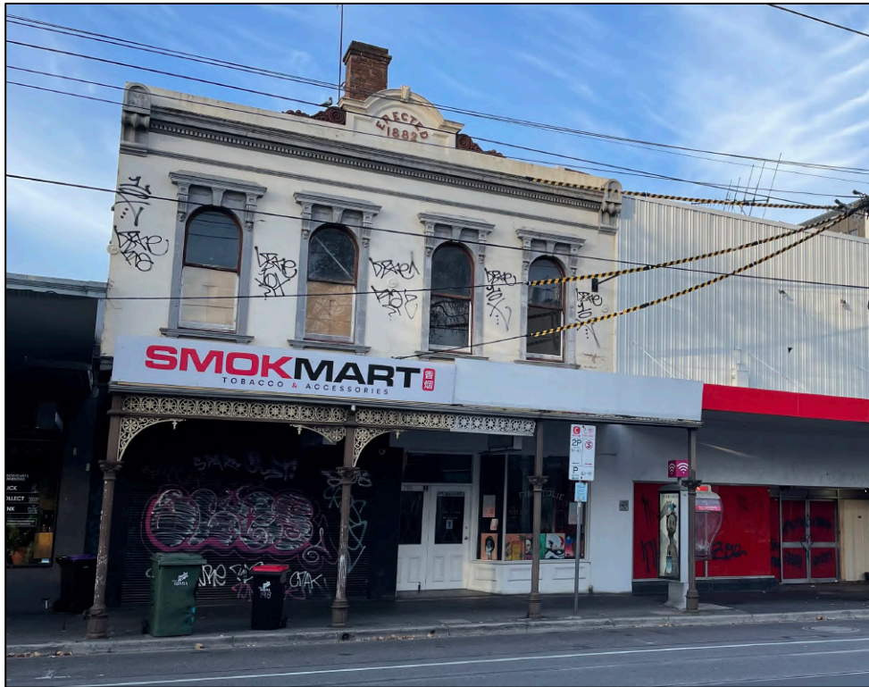
Figure 8 198-200 Swan Street, highlighting the rendered upper level façade.
