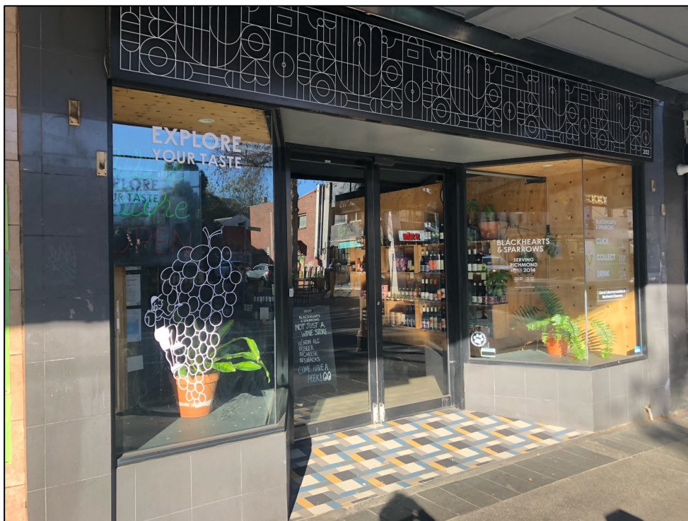
Figure 7 The shopfront of 202 Swan Street. It is identified as non-contributory, with an altered, early 20 th century character.
