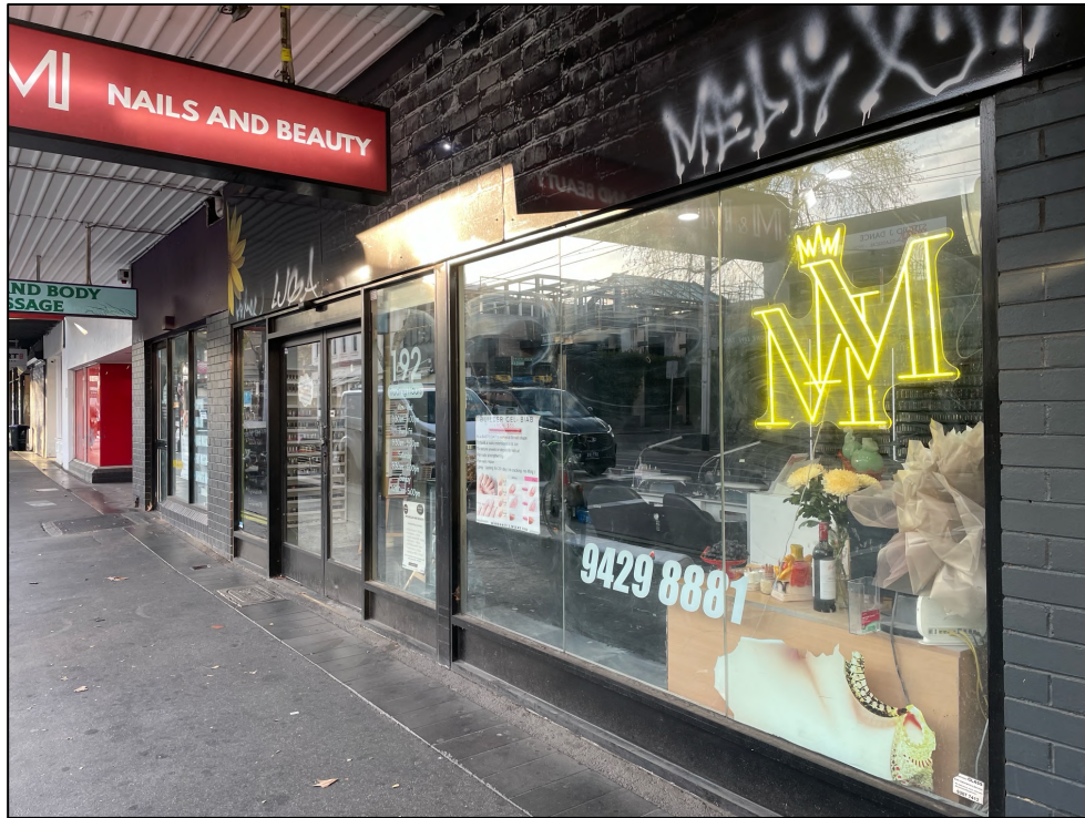
Figure 10 The far western modern shopfront associated with 188-190 and 192 Swan Street, noting the shopfront is numbered only as 192.
