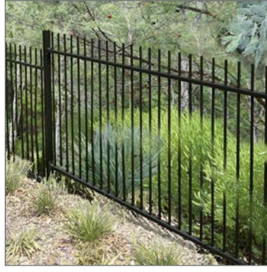
SECURE OPEN PALISADE FENCE
