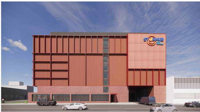
Figure 16 Barkly Avenue facade showing sign in top right corner
