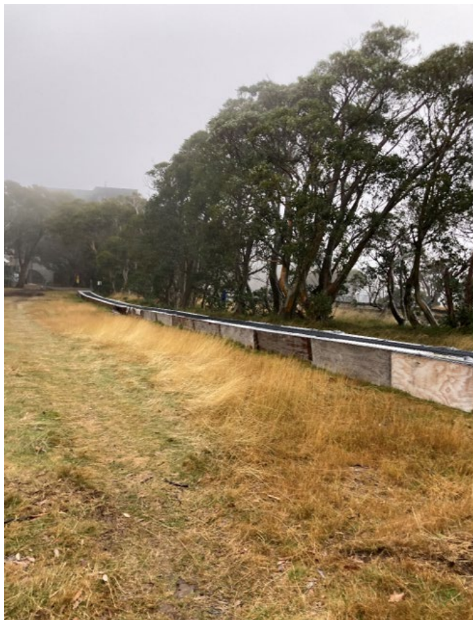
Figure 5: Photo taken of Magic Forest 1 magic carpet lift facing south-east (Source: Site photos taken by DTP officers during site inspection on 28 April 2023)
