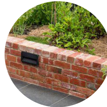
Brick retaining wall
