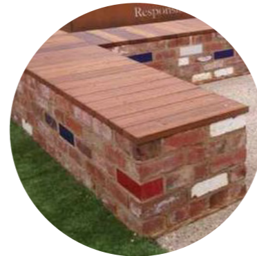
Brick paving and seats with brick base and timber battens
