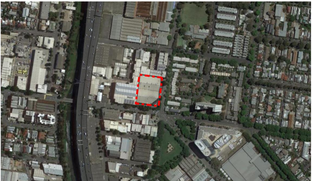
Figure 1 - Pre-existing sites at 218-246 Macaulay Road, North Melbourne.
