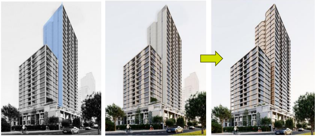
Figure 25: Material detail and extruded horizontal slab edges be reinstated in the book ends
