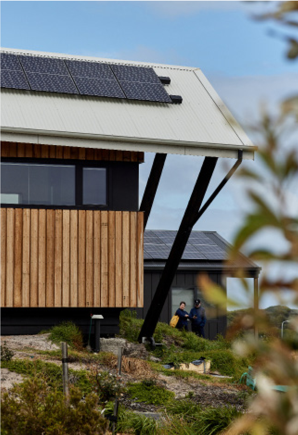
Rooftop Solar PV at Cape Paterson. Photography by Kim Landy.
