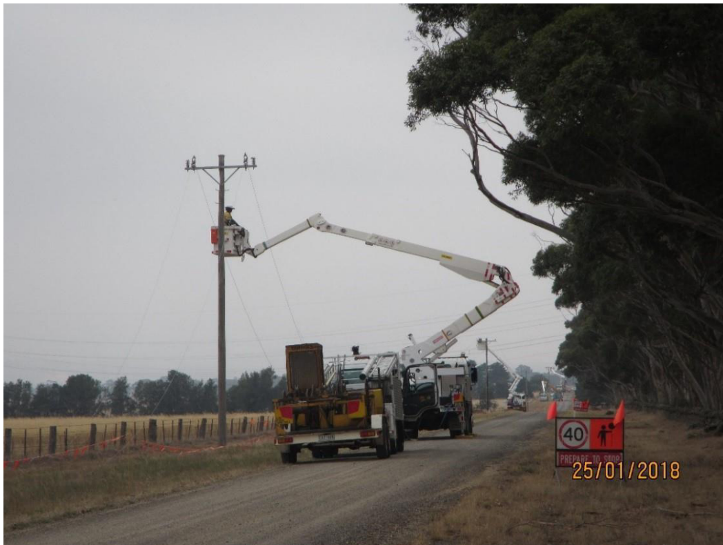
Figure 5. Example of contractors working on the new or replacement installation. Note the truck is still in the road carriageway
