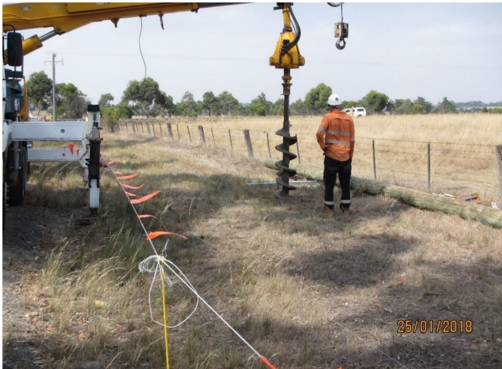
Figure 3. Example of hole being augured via arm from truck (note in this example the roadside vegetation was deemed to be native in places and fencing was set up to keep the truck from the shoulder)
