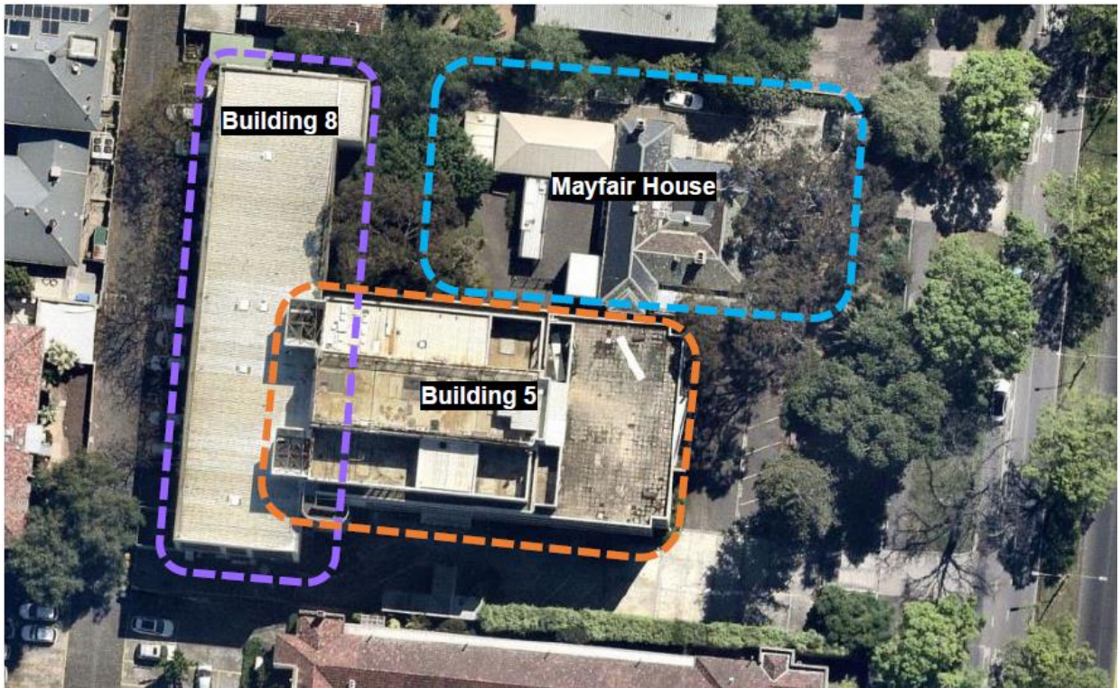
Figure 1 Existing site buildings labelled
