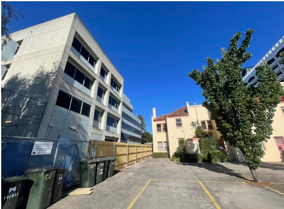
Figure 20 Southern site boundary and adjoining apartments at 321 Royal Parade
